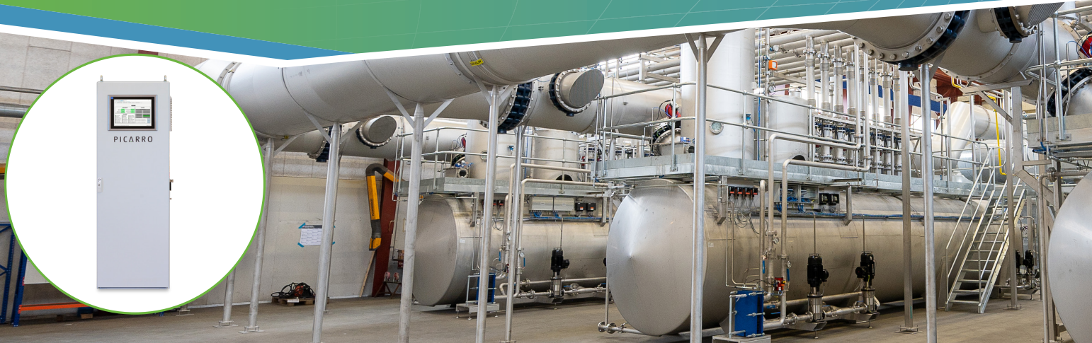
Figure 1: LESNI EO Catalytic Abatement Plant (EO CAP), with Picarro Continuous Emissions Monitoring System (CEMS) inset.
