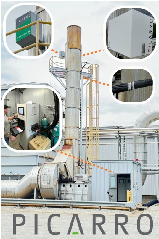
Figure 3: The Picarro EtO CEMS, showing the cabinet itself (left middle), flow probe (left top), sample probe (right top) and heated umbilical (right middle).
