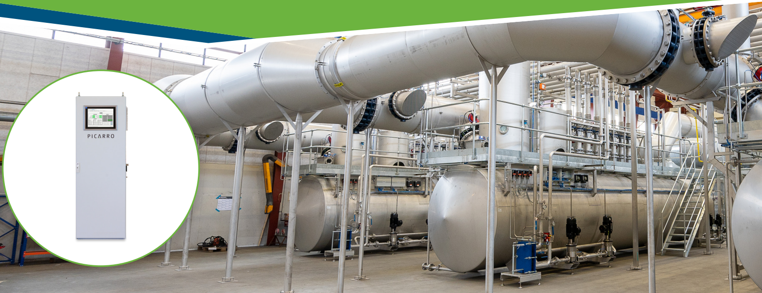
Figure 1: LESNI EO Catalytic Abatement Plant (EO CAP), with Picarro Continuous Emissions Monitoring System (CEMS) inset.
