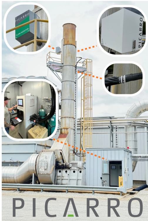
Figure 5: The Picarro EtO CEMS. State-of-the-art Picarro CRDS technology sits within a NEMA-12 (or better) industrial enclosure, with an umbilical connecting the system to the stack, where flow monitoring and sample probes feed back essential parameters, sample and calibration gases to enable real-time monitoring of concentrations and computation of mass emissions.
