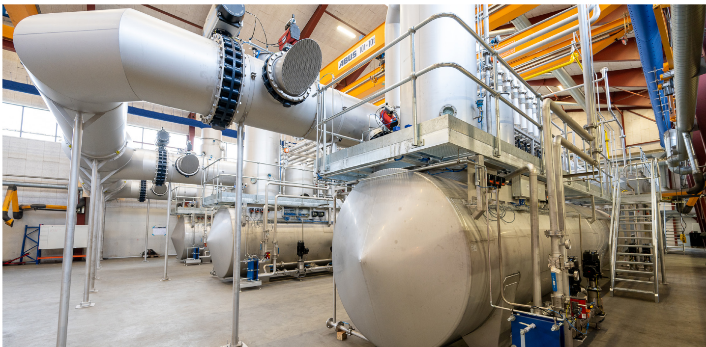
Figure 3: One configuration of a LESNI EO CAP, which Picarro Technology shows abates EtO Emissions well beyond the new NESHAP requirements promulgated by the US EPA. Featured are the balancer water tank (bottom center), scrubber column (upper center- left), and various process gas ducting (top right, middle left). The CatOx beds can be seen as a silver rectangle just above the burner in the middle right of the background.
