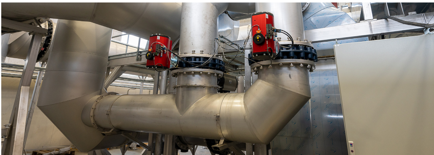
Figure 2: Ducting around a LESNI EO CAP showing the sophisticated management of process air by valving.
